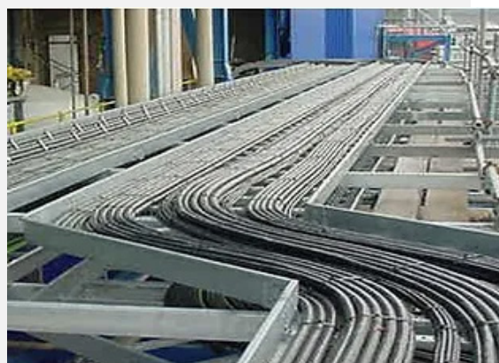
Indoor Fiber Cabling
