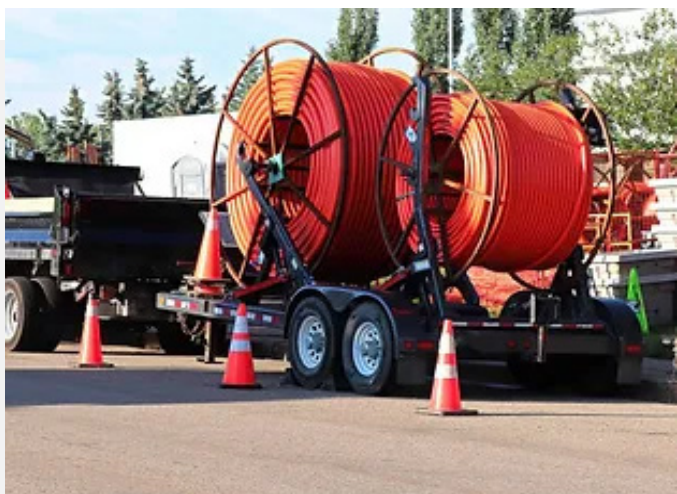
Outdoor Fiber Cabling
